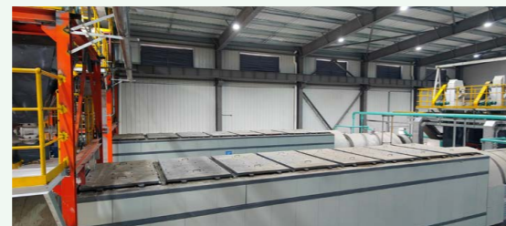
Ningbo Haijing fly ash medium-low temperature pyrolysis EPC project
