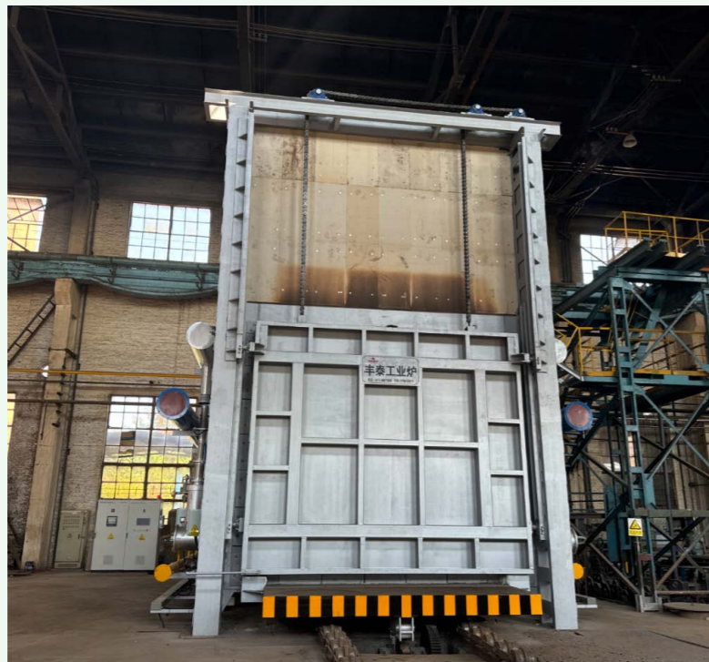
Furnace upgrading project
