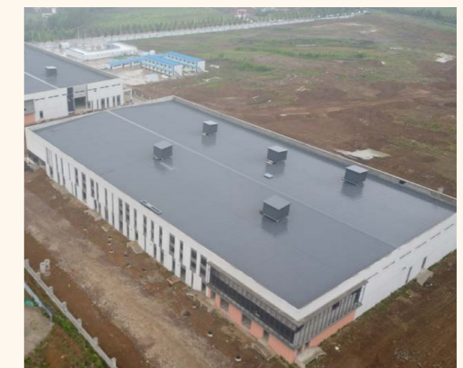
Rural revitalization livestock farming demonstration base infrastructure project in Dongfeng County
