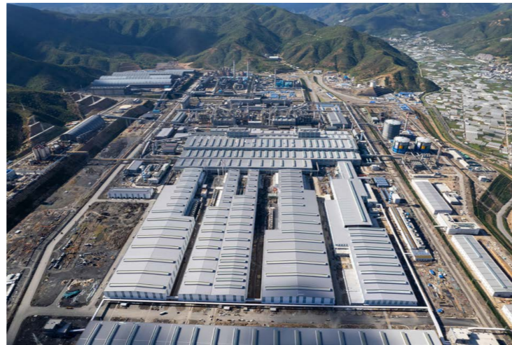
Yunnan Yukun Steel Project
