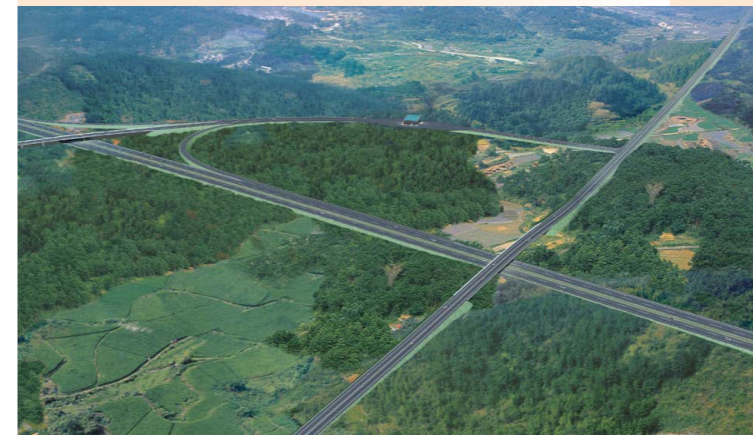
Liuzhou Highway Bypass Project (Luocheng-Liucheng-Luzhai Section)
