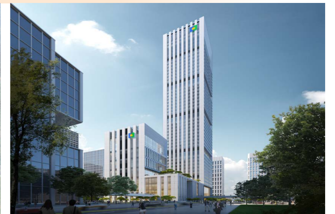
Hengli Group Shenzhen Bay super headquarters base main project
