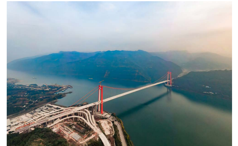
Chongqing Jianglong Expressway rejuvenation Yangtze River Bridge project
