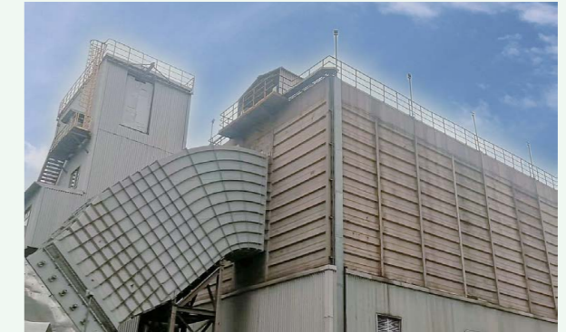
The EMC energy-saving renovation for the dust removal system at the Baoshan steel-making plant
