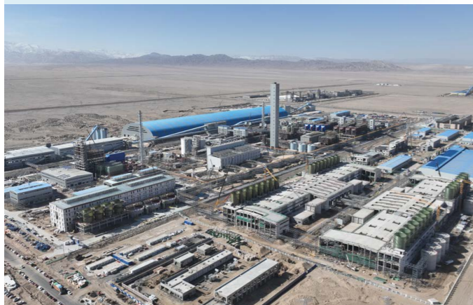
Xinjiang Huoshaoyun Lead-Zinc Smelting Project
