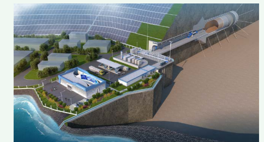
50,000Nm 3 horizontal tunnel underground hydrogen storage system
