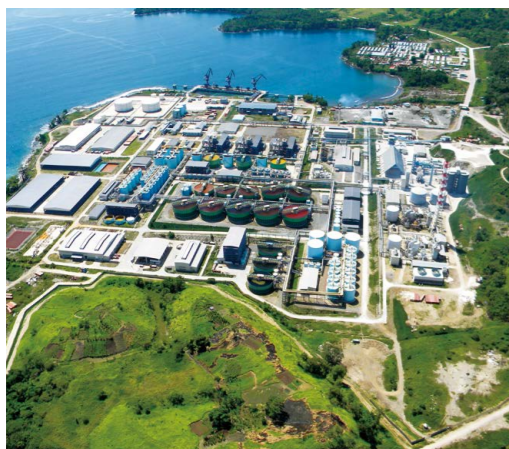
Ramu Nickel-Cobalt Mine Project, Papua New Guinea
