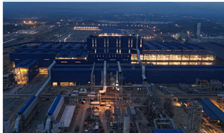
Vietnam Hoa Phat Dung Quat Steel Plant Project
