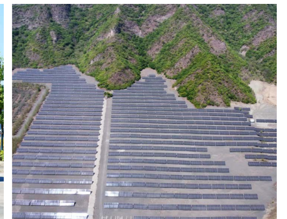
South-to-North Water Diversion New Energy Kuancheng Ground-Based Distributed Photovoltaic Project
